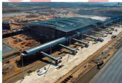
King Shaka International Airport
